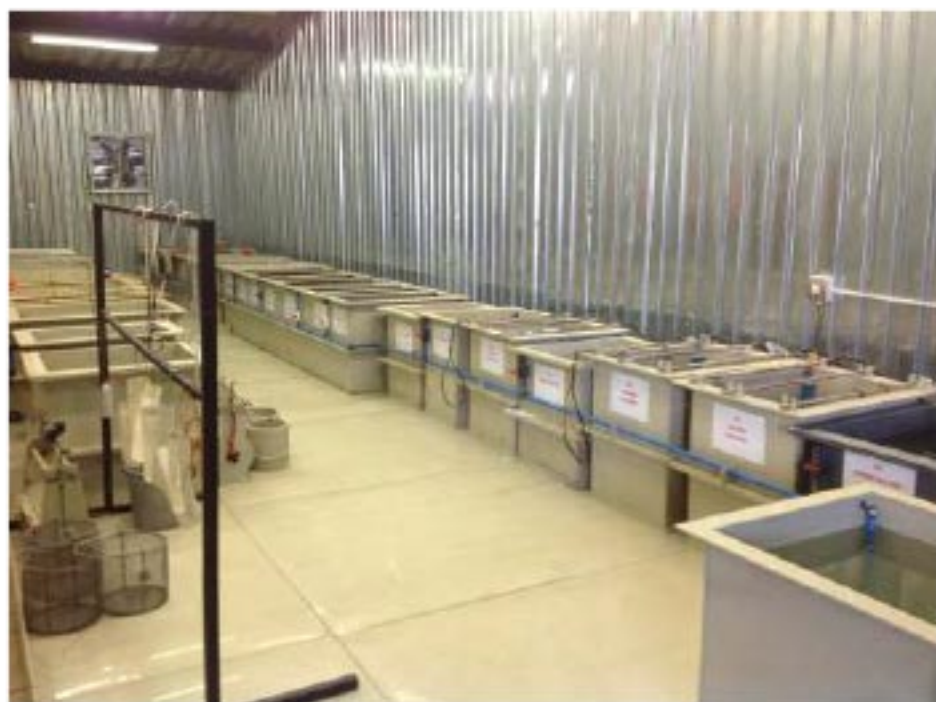
Installation of the new plating plant
